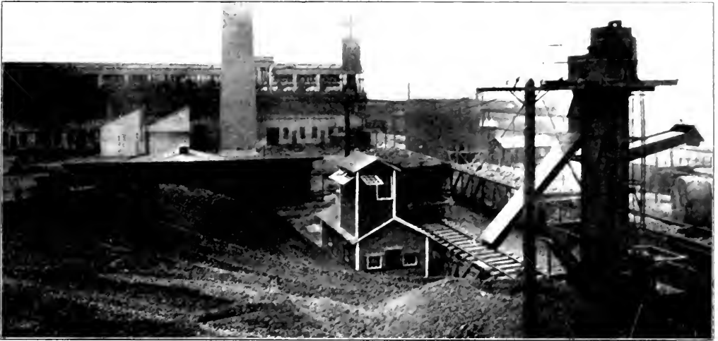
FIG. 2. COAL IS MOVED BY CARS FROM BARGES TO AN ELEVATOR AND DUMPED TO THE STORAGE.
